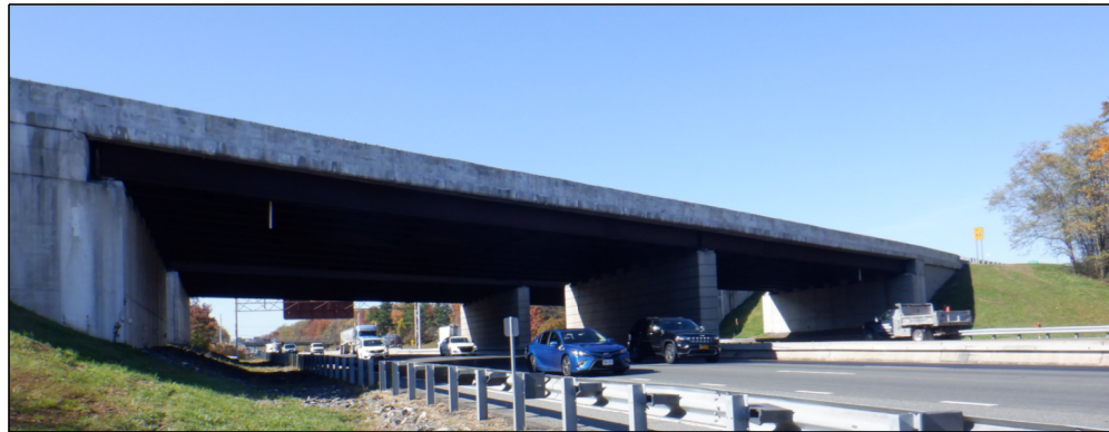
EAST ELEVATION VIEW A
