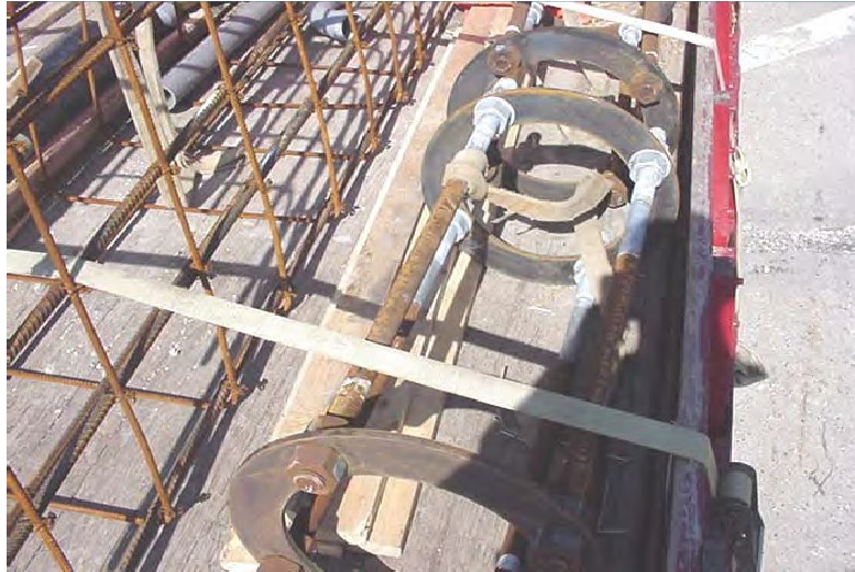
Figure 1. Four Anchor Rod Group in a Template.
