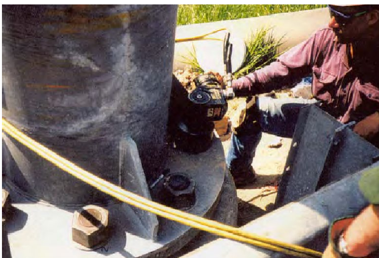
Figure 3. A Hydraulic Torque Wrench Tightening Anchor Rod Nuts to Achieve Needed Rotation.
