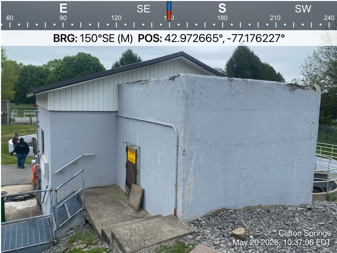
Photo 1: exterior wet well hatch
