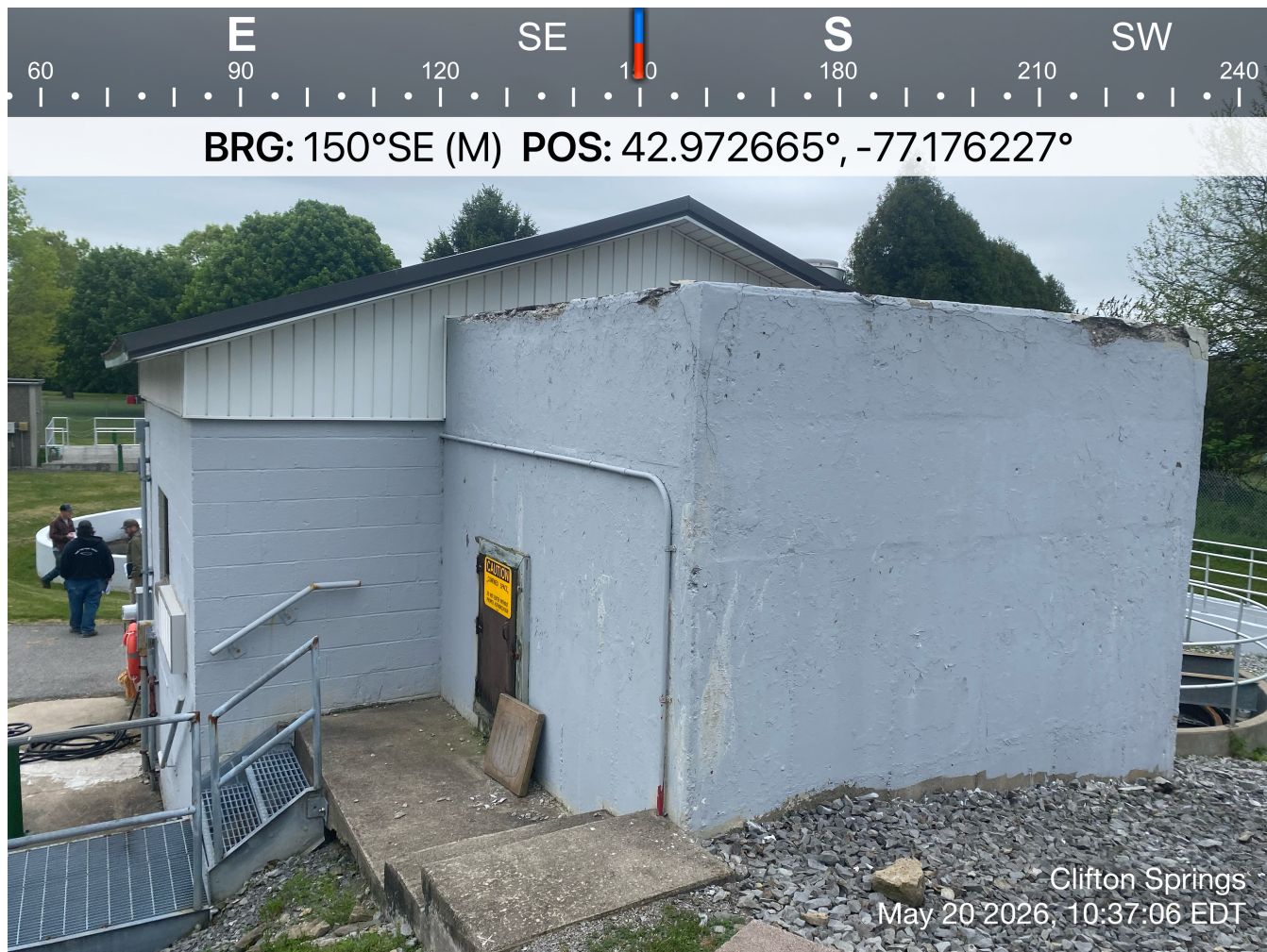
Photo 1: exterior wet well hatch
